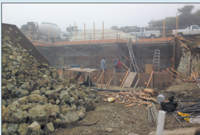
Contractor photos document the process: from top left, the old house, which was deconstructed for salvage; a tractor with a shifter was used to sort rocks for later use in retaining walls and landscaping; laying out the foundation of the upper floor; builders cut about 12 feet back into the hill in order to construct the lower floor; the house takes shape.
